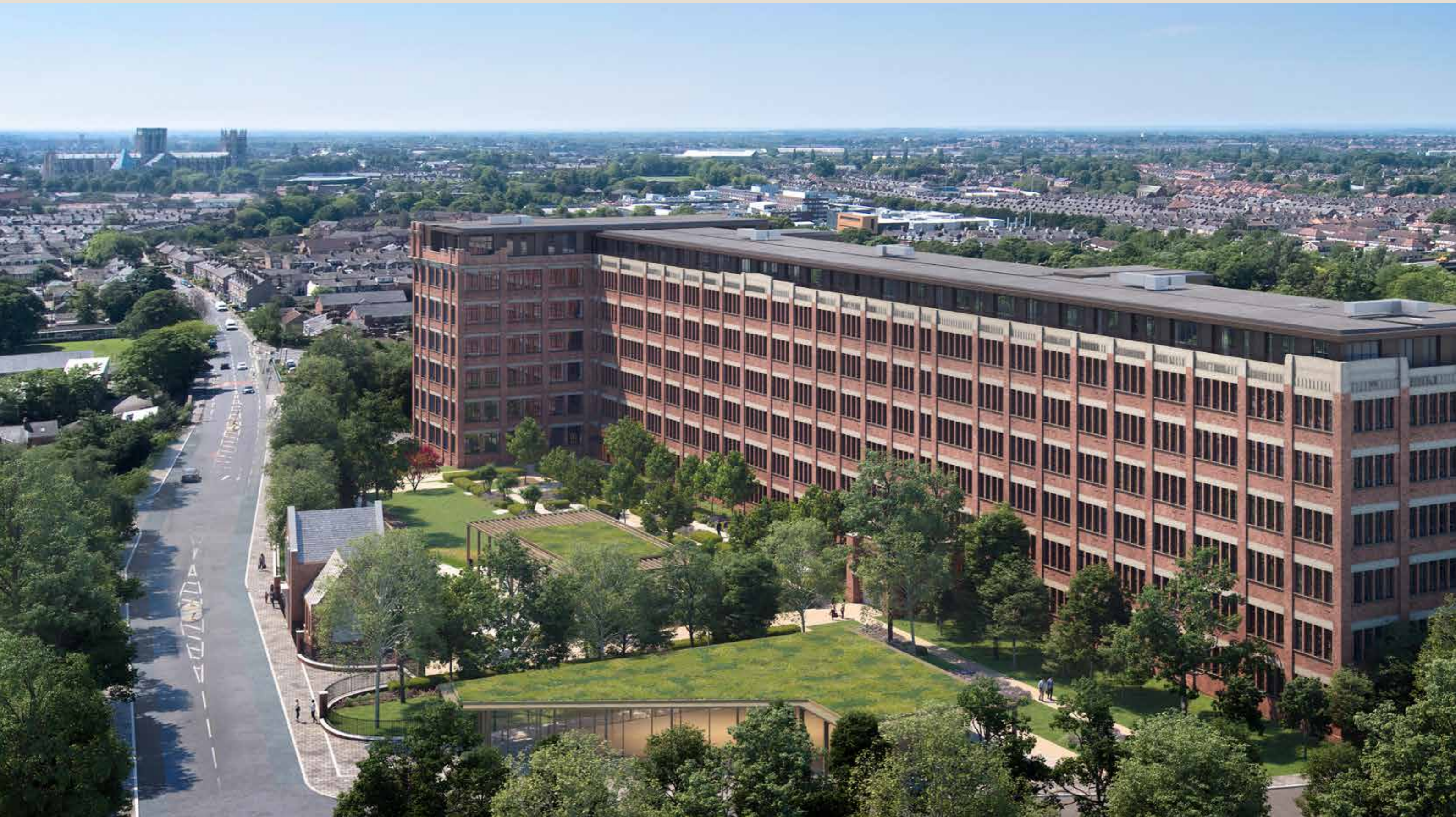
THE HAXBY ROAD VIEW DETAILING THE FORMER LIBRARY NOW CONCIERGE, CONVENIENCE STORE AND CAFE
